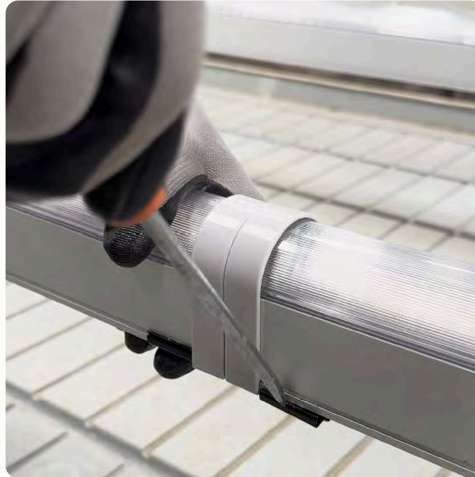
Fig 10. Removal of Interconnection Clips
