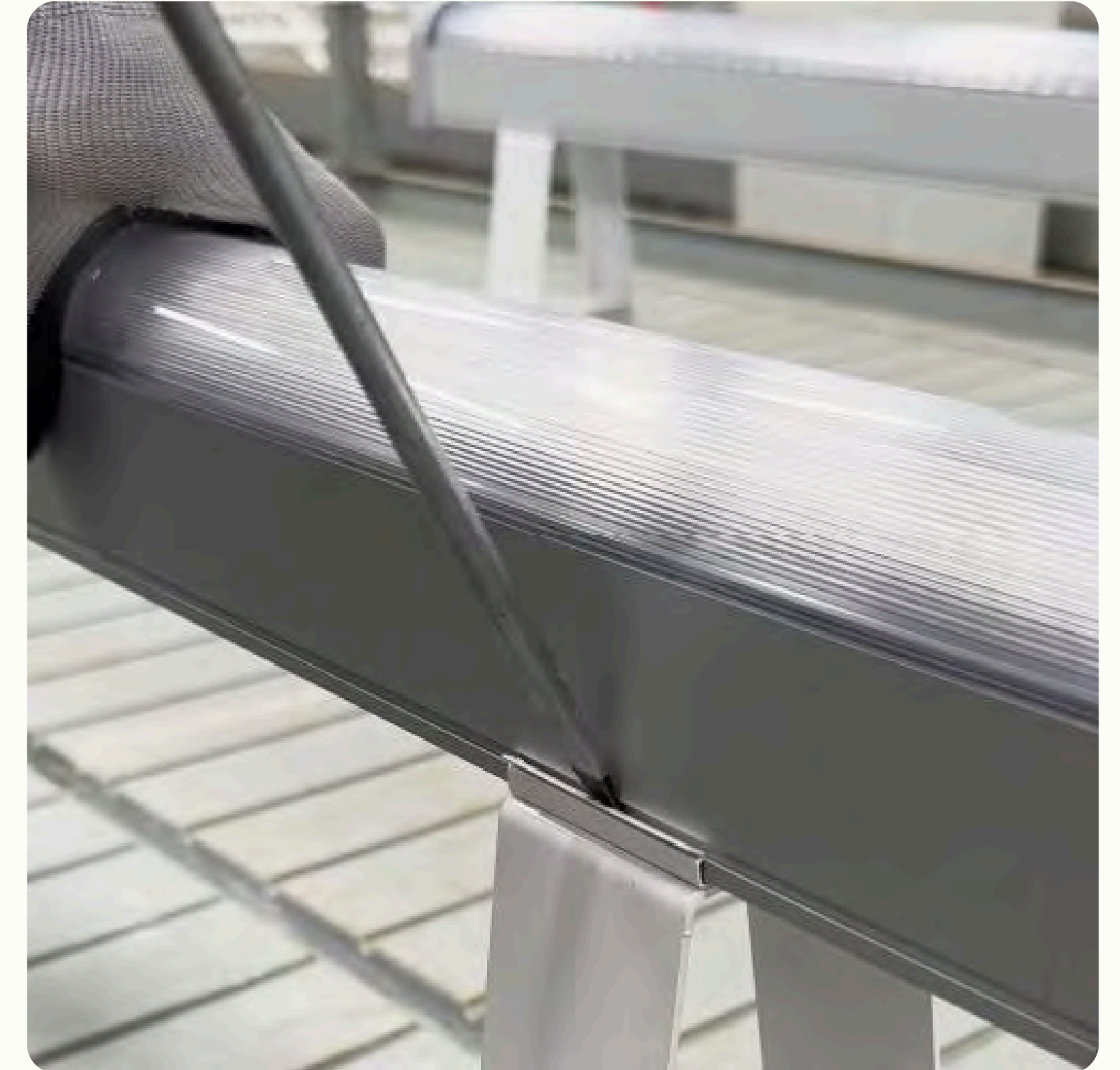
Fig 11. Disengage lights from Mounting Brackets
