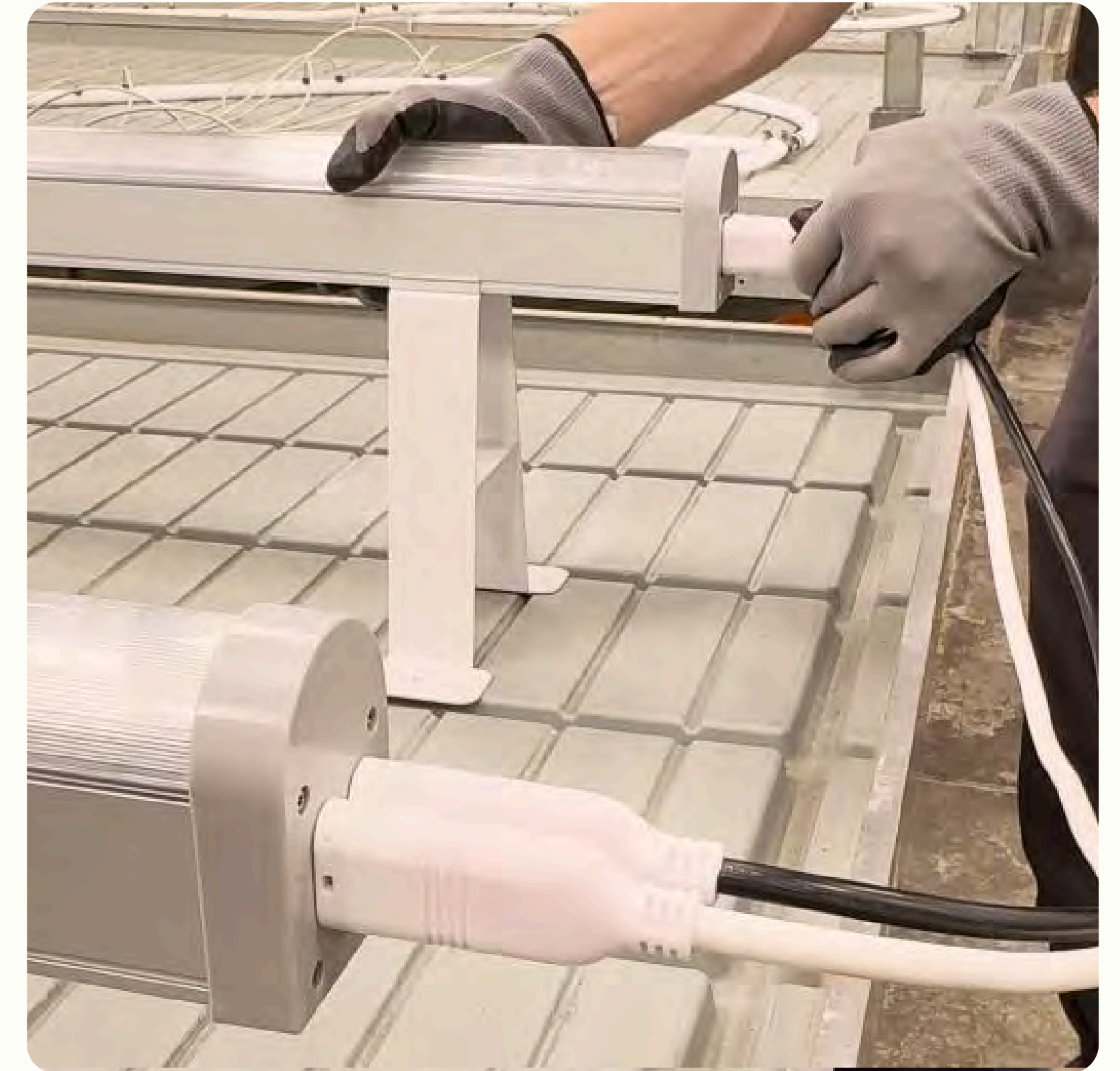
Fig 6. Dimming connections
