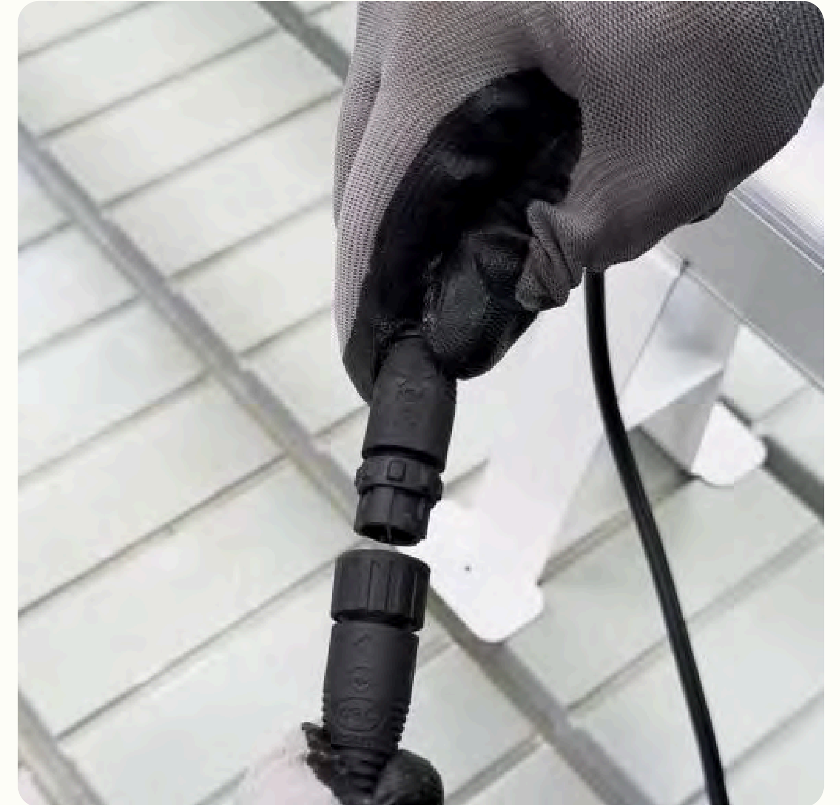
Fig 8. Dimming Quick Connect cable connection
